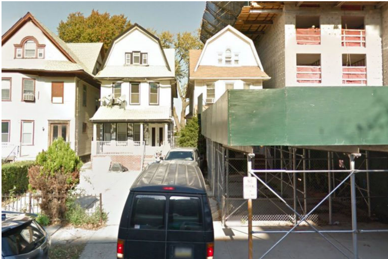
Pre-demolition 323–325 Lenox Road. Image via Google Maps.
